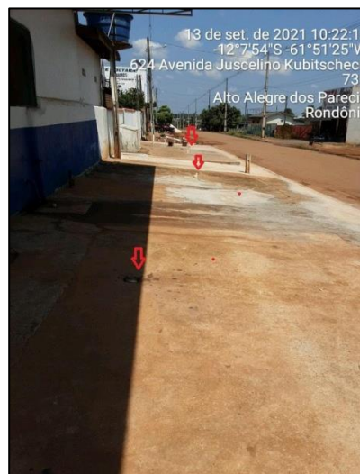
Fossa Rudimentar – Av. Juscelino Kubitschek. 12°07'54.00''S e 61°51'25.00''W.
