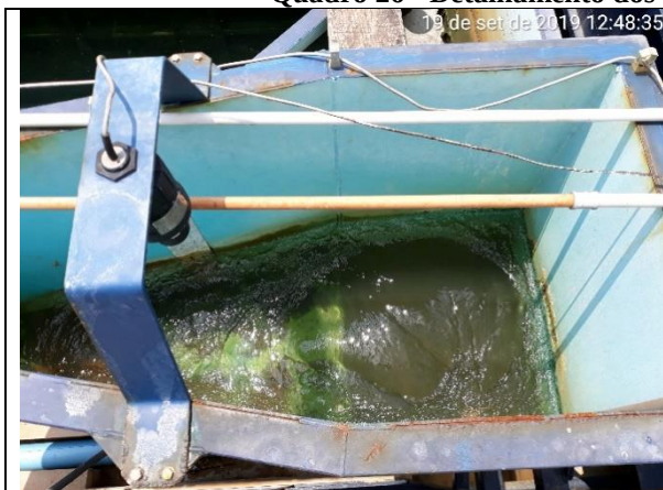
Calha Parshal 9 polegadas Q= 55,0 L/s
