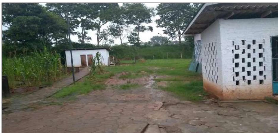
Figura 183 - Abrigo no hospital municipal
