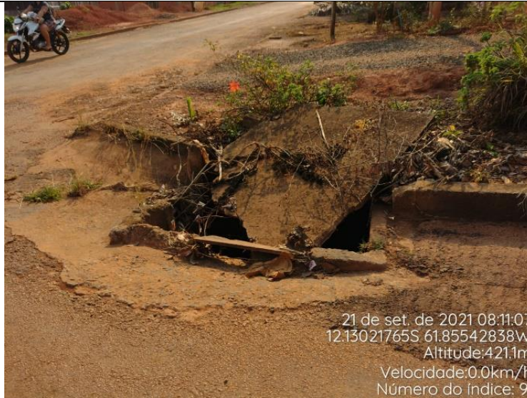
Rua Marechal Rondon
